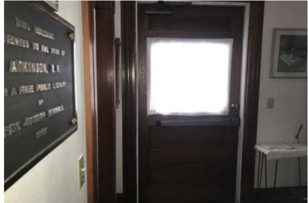
#20 EXTERIOR DOOR, WOOD SOLID-CORE
