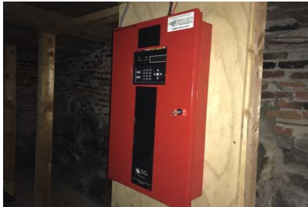
#27 FIRE ALARM CONTROL PANEL
