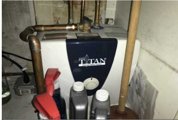
#25 WATER HEATER, ELECTRIC
