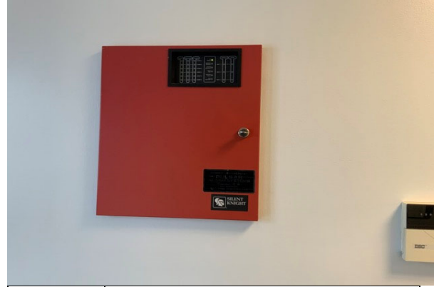
#26 FIRE ALARM CONTROL PANEL, ADDRESSABLE
