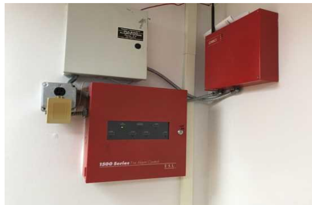
#30 FIRE ALARM CONTROL PANEL
