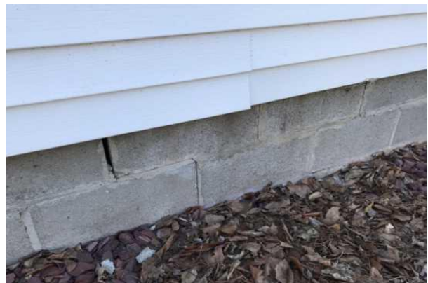
#18 CMU SUBSTRUCTURE, LOOSE MORTAR JOINTS
