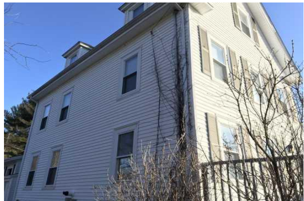
#16 EXTERIOR WALL, VINYL SIDING
