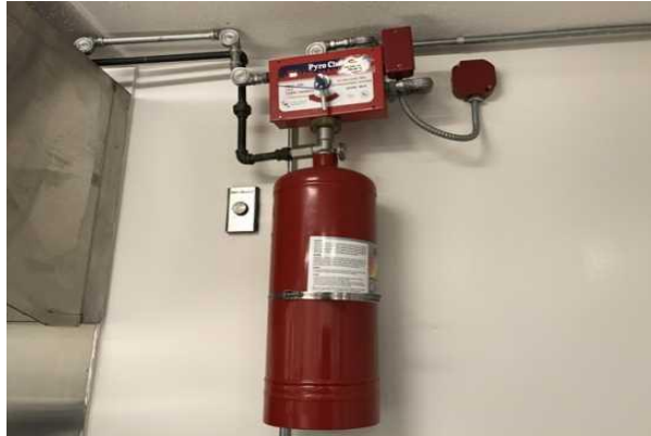
#31 FIRE SUPPRESSION SYSTEM, KITCHEN HOOD
