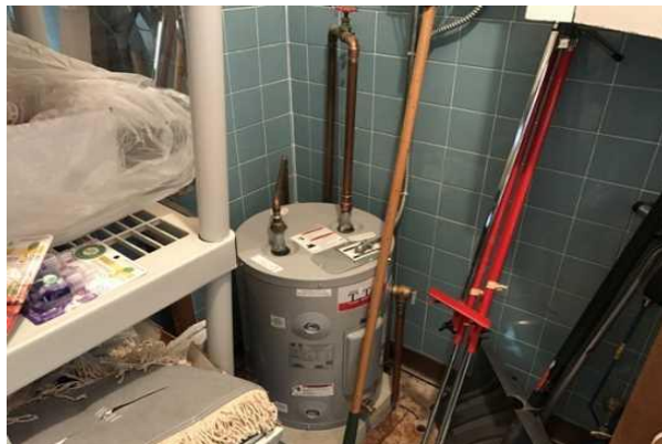
#27 WATER HEATER, ELECTRIC
